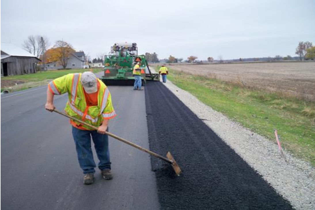
Figure 45 Warm Mix Asphalt Application
