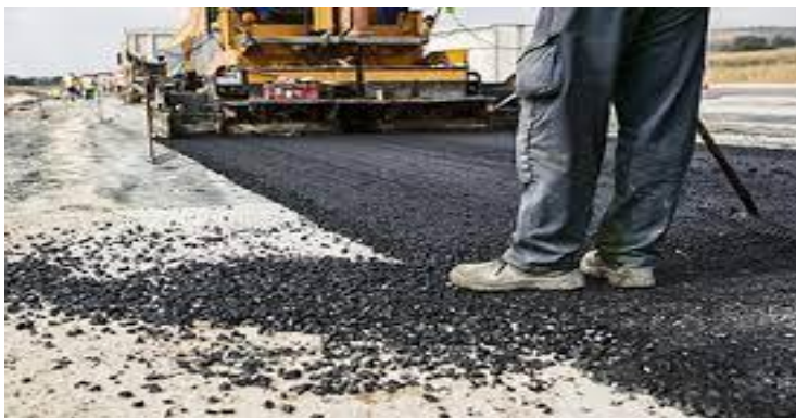
Figure 42 Sand- Asphalt Mix Application
