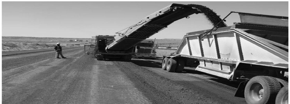
Figure 50 Milling of Reclaimed Asphalt Surface
