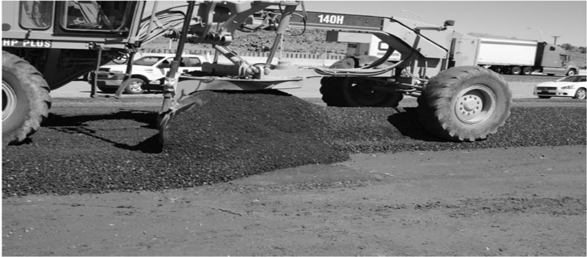
Figure 54 RAP-Mixed Base Course in an Interstate Pavement in New Mexico
